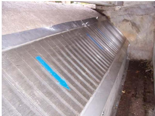
Figure 1 –Curb Inlet Installation
