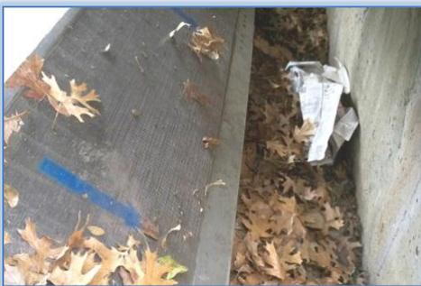
Vector control is not an issue and bacterial growth is significantly impeded because the captured debris remains dry. No special handling techniques are required for debris removal and can be disposed as ordinary municipal waste.
