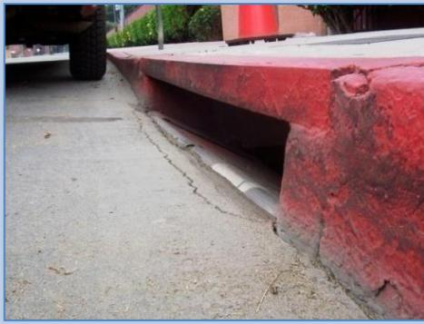
The COANDA Approach Plate, barely visible, fits snug against the curb inlet opening so as not to impede water flow or be exposed to traffic.
