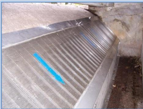
The interior of the curb inlet shows the COANDA screen on the right, through which all water passes, and the large debris compartment on the left. Optional treatment is provided underneath the screens.
